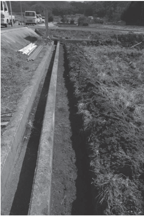
②基礎の根堀
